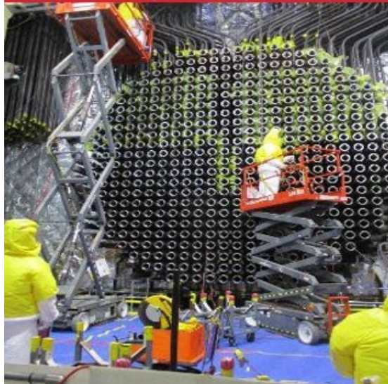
Fuel Channel & Feeder Replacements (RFR & FCFR)
