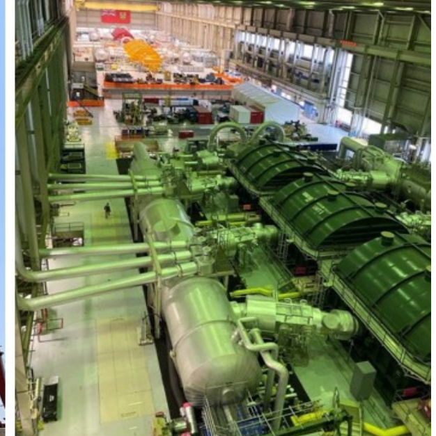
Turbine Generator Refurbishment (TGR)
