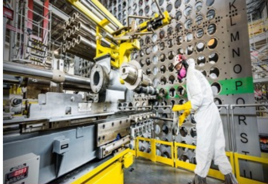
Fuel Channel & Feeder Replacements (RFR & FCFR)
