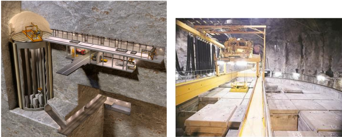
Figure 8-11. The silo for disposal of the most active LLW in SFR
