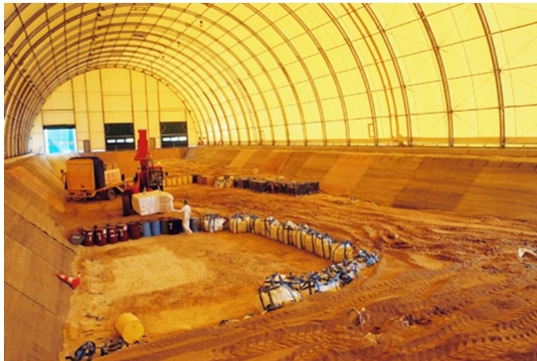
Figure 8-2. Disposal of VLLW waste at the special disposal facility for such waste at Morvilliers, France. (Courtesy of Andra)
