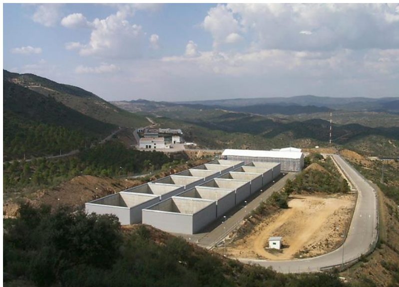
Figure 8-5. Aerial view of the El Cabril disposal facility in Spain. (Courtesy of Enresa)
