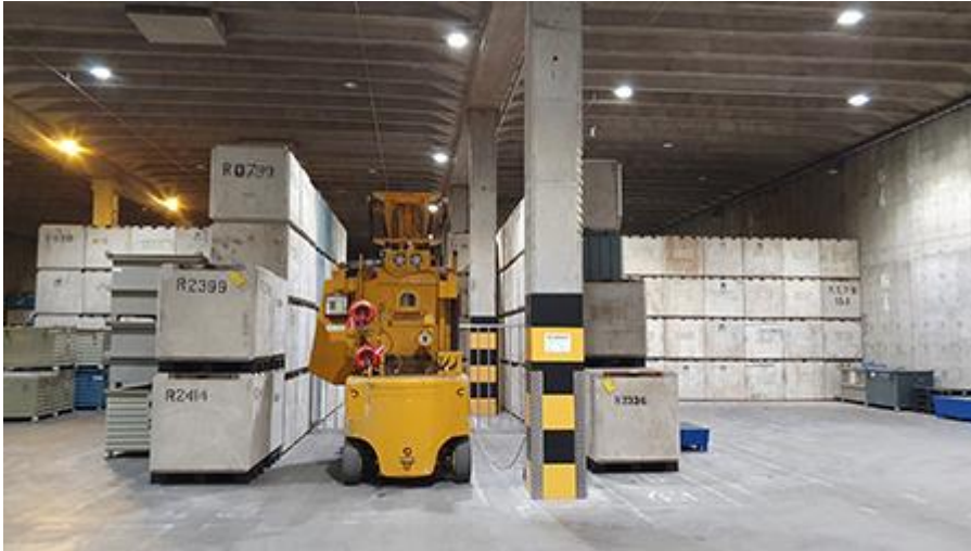
Figure 7-4. Shielded fork lift truck for transport of RW packages in Ringhals, Sweden.
