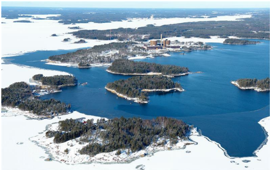
Figure 9. Aerial photo of the Loviisa NPP in winter 2009. 47
