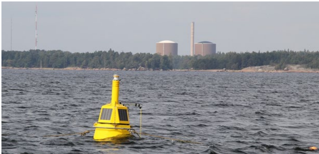
Figure 8. Additional sea water measurement buoy in the sea area outside of the Loviisa NPP. 46
