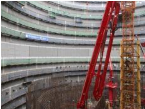
Photographing during placing concrete
